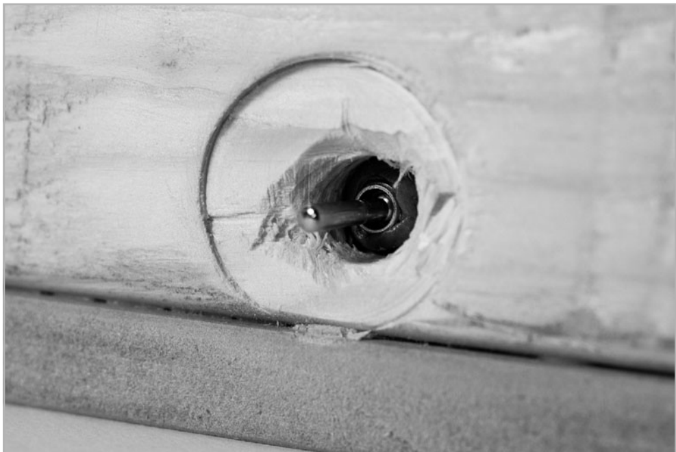
FIGURE 10-10 A view of the switch from the outside
